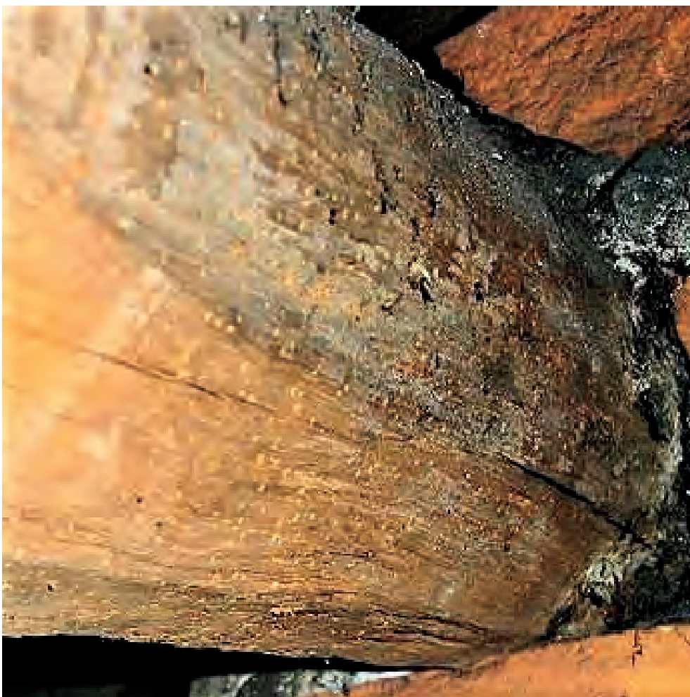
Beetle attack to the outer sapwood of a beam
