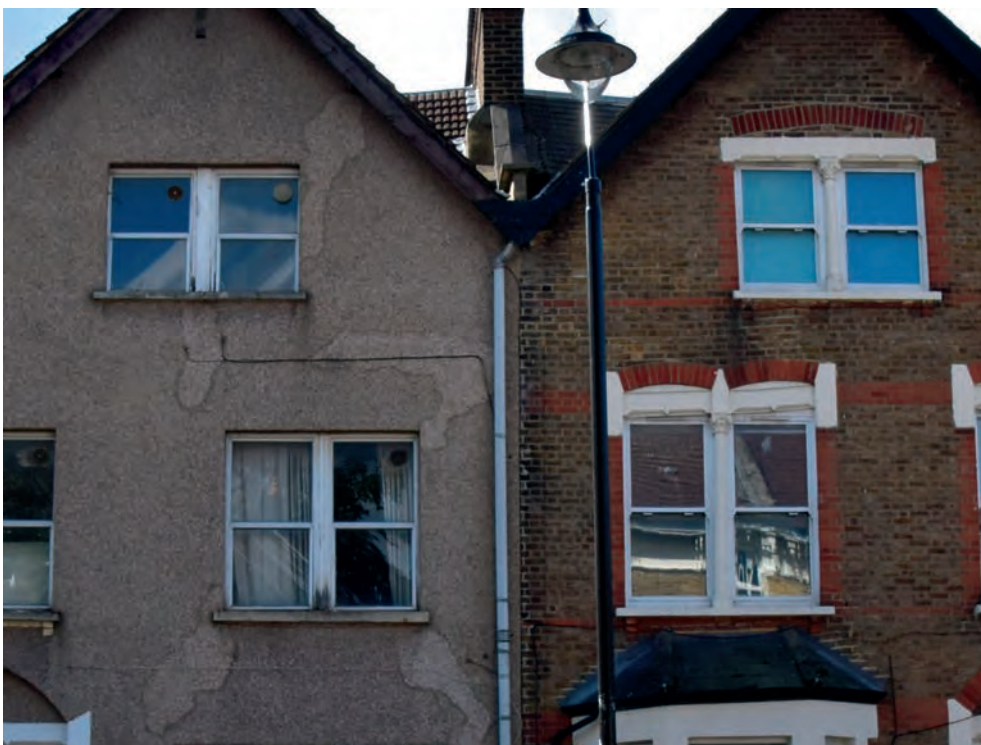
Modern pebbledash render alongside original brickwork.
