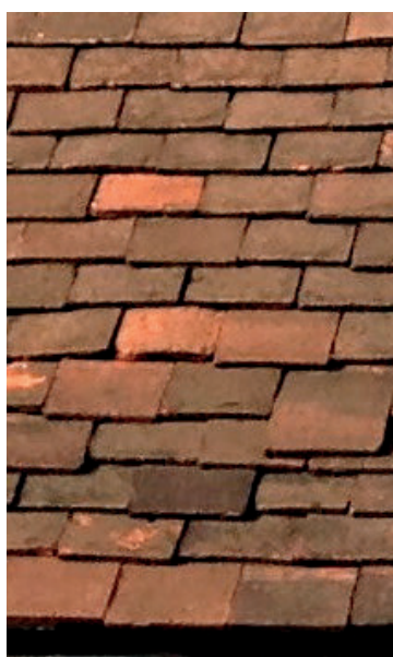
(L) Missing and slipped slates allowing rain to get in.
