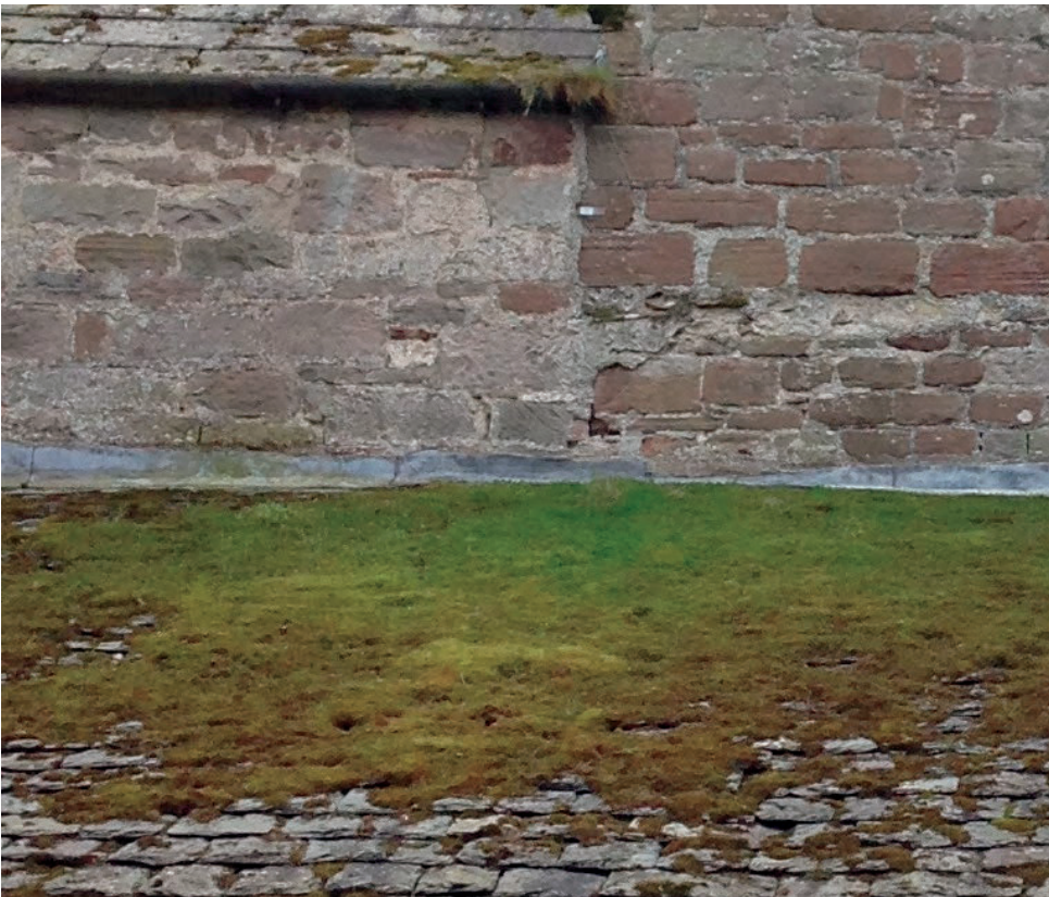
Excessive moss growth on roofs.
