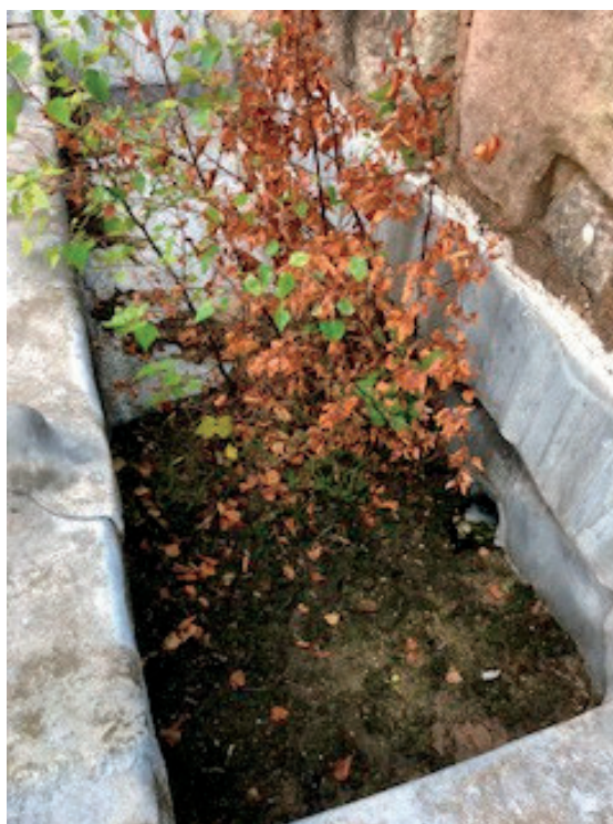
(R) A tree sapling allowed to grow in a parapet gutter.
