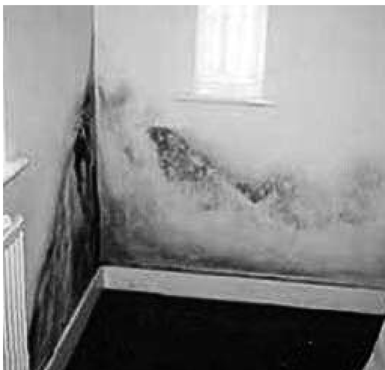
Mould growth, often an indication of condensation
