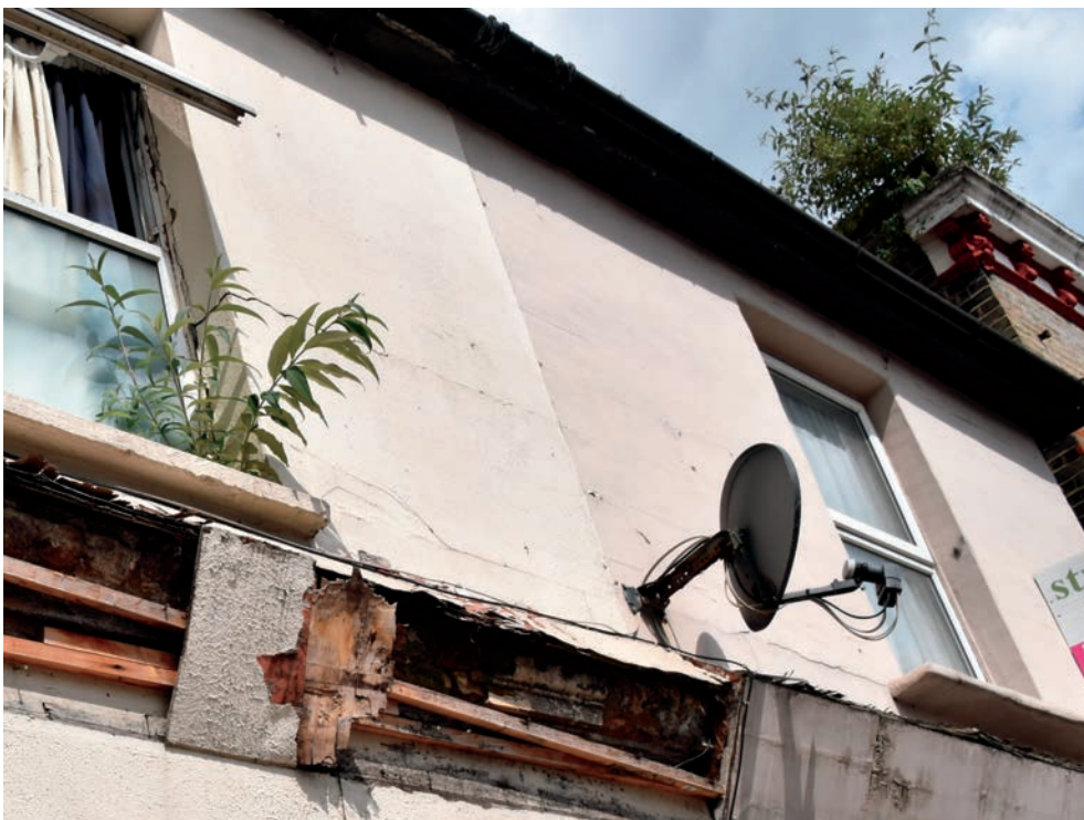
Decay caused by lack of maintenance.
