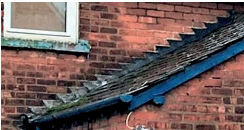
A stepped lead flashing at the abutment of a roof and wall.
