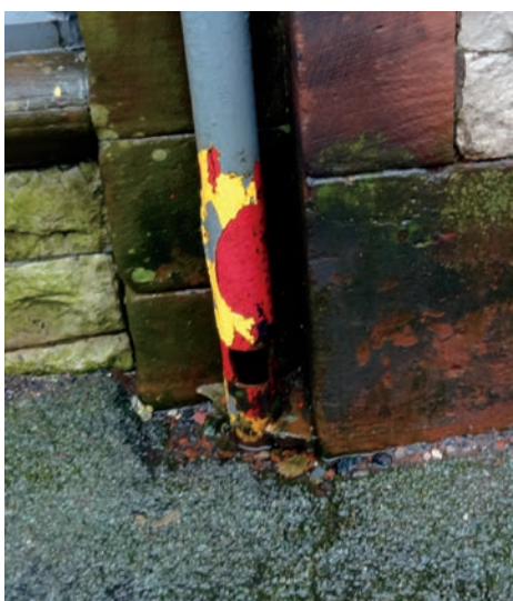
(L) A blocked rainwater gulley not draining away.
